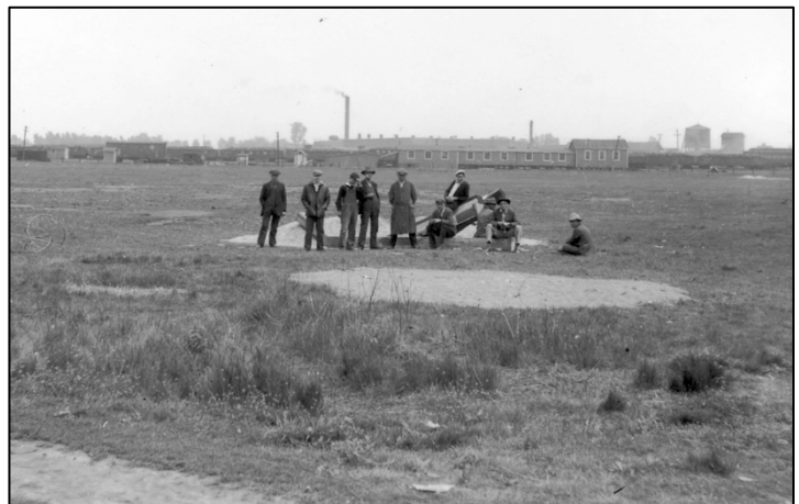
Groundbreaking at the mill site, looking northeast. May 1929.
