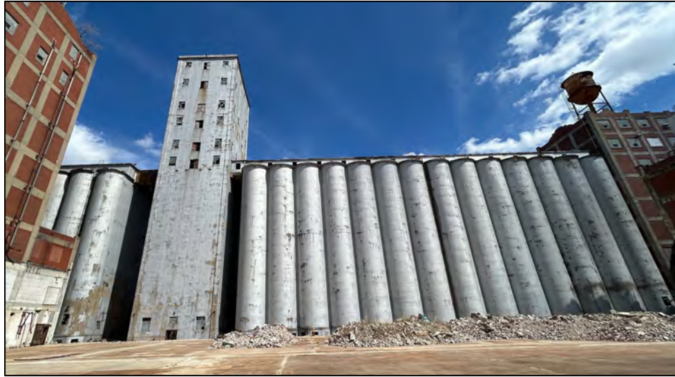
Grain silos and Head House, view from the west. Demolished remains of Warehouse #1 in foreground.
