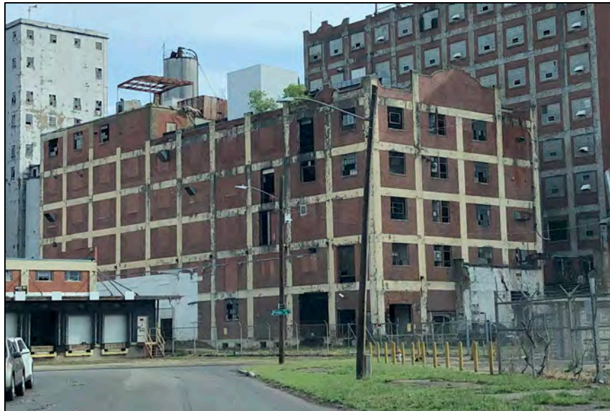
Exterior view of the Grocery Mix Building, from the southwest.
