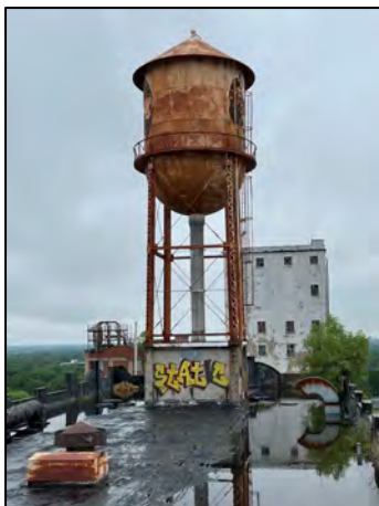
Water tower atop A-B Mill.
