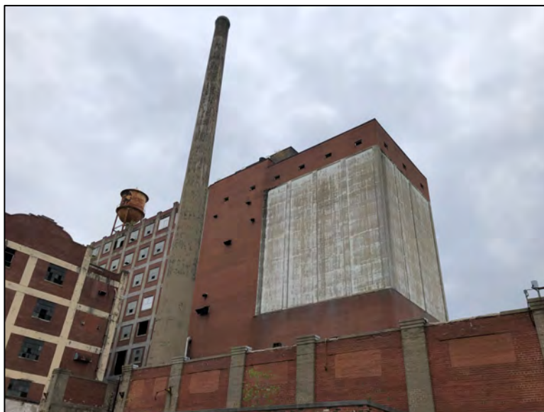
The Turbo / Bulk Storage Building, on the south end of the A-B Mill.
