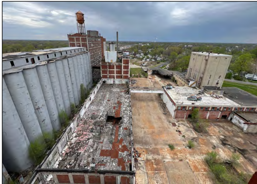
Aerial view (from the north) of Warehouse #1 in late 2022. Roof removed prior to 2015. (Photo: Chris Richmond)
