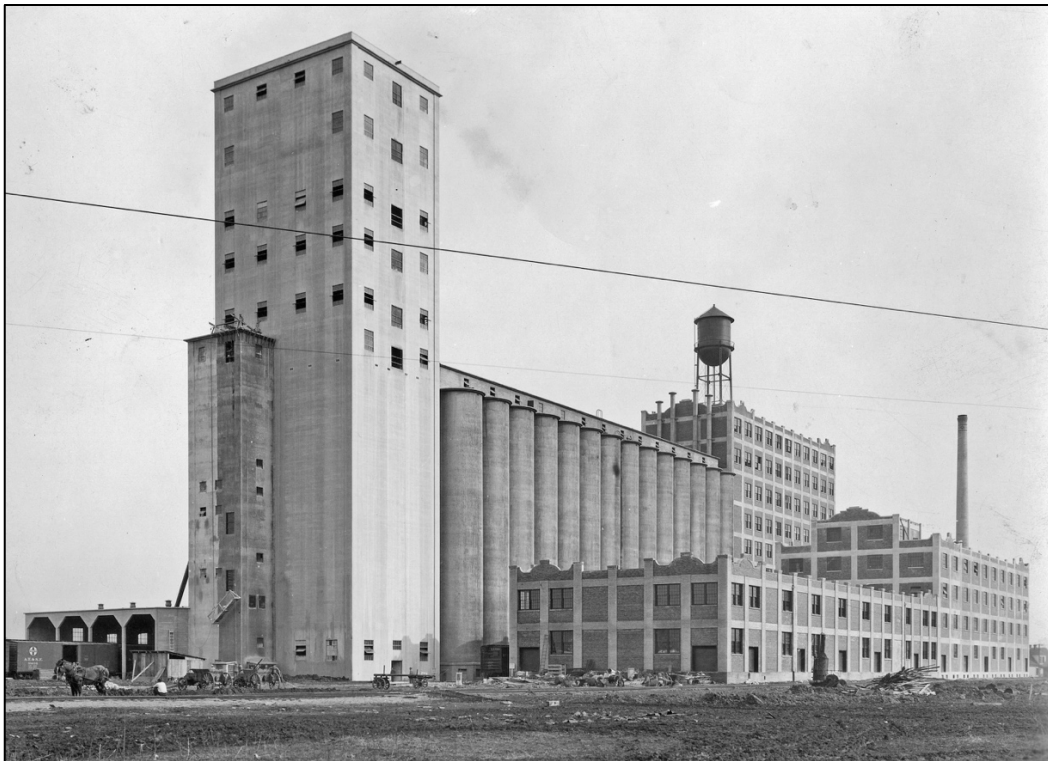
1930 view (from the northwest) of nearly-completed first phase of mill.
