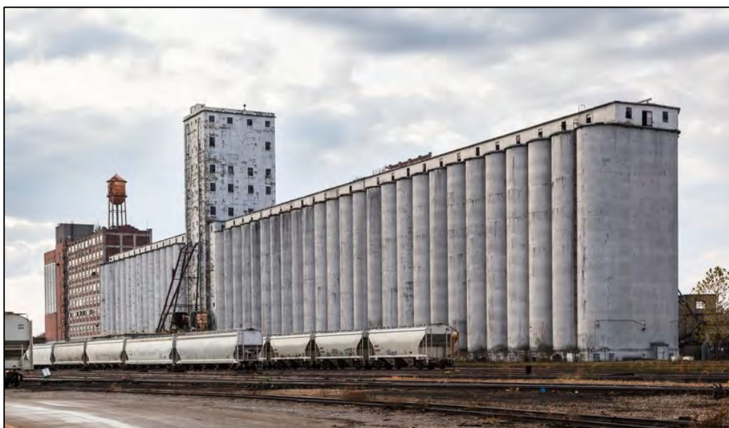
Grain silos and Head House, view from the northeast. (Photo: Ben Halpern)
