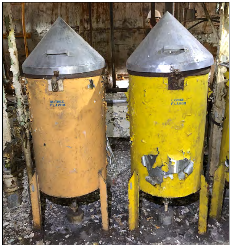
Flavoring tanks on 4 th floor of Bakery Tower.
