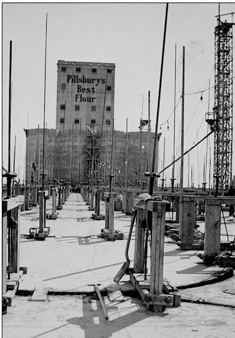
Head House completed, silos under construction (view to north).
