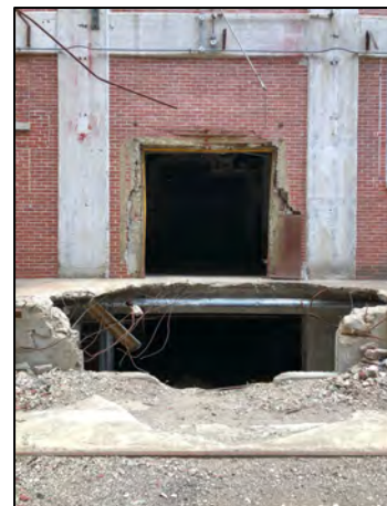
Damage to the A-B Mill from large-scale metals salvage.
