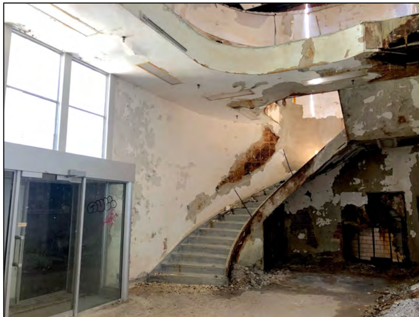
Lobby and main public staircase to administrative offices.
