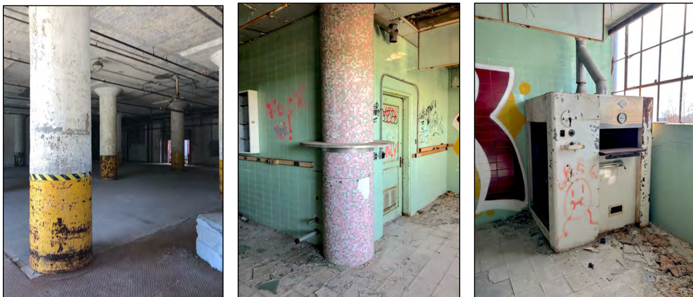
First floor view (left), and fourth floor test kitchen (middle, right) in Grocery Mix Building.
